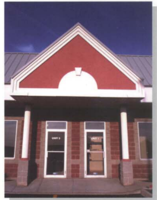
COMMERCIAL BLDG. 25 STRUCT CRT. CAMBRIDGE, ONT.
